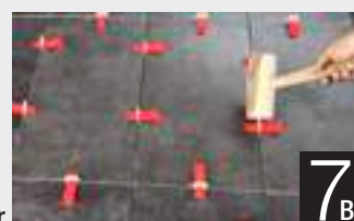
7B Or simply Remove Wedges with a Mallet
