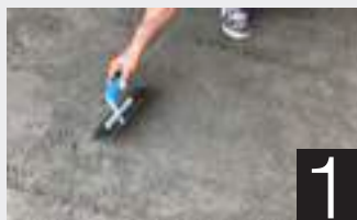
1 Apply Tile Glue / Cement
