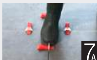
7A Simply Remove Wedges with a kick
