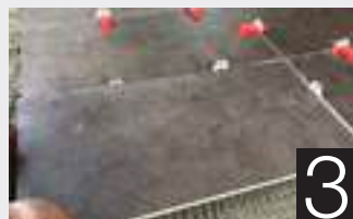
3 Place the other Tile over the other end of Tile Spacer
