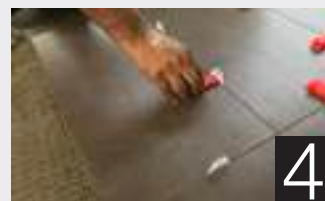
4 Insert Wedge into the Tile Spacer
