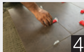
Insert Wedge into the Tile Spacer
