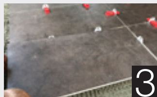
Place the other Tile over the other end of Tile Spacer
