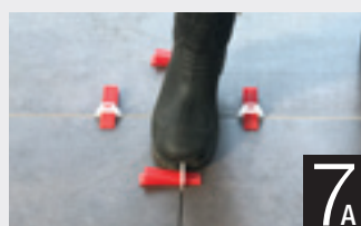
7A Simply Remove Wedges with a kick
